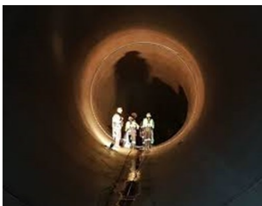
Inside a penstock
